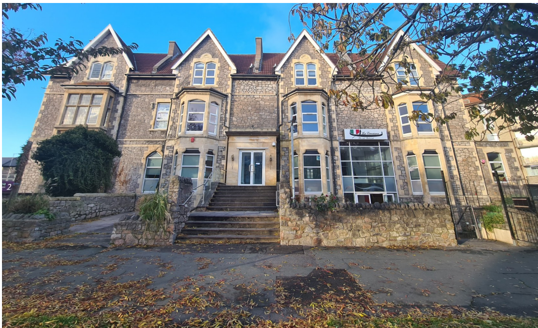
Indicative image of a fitted office in the building
