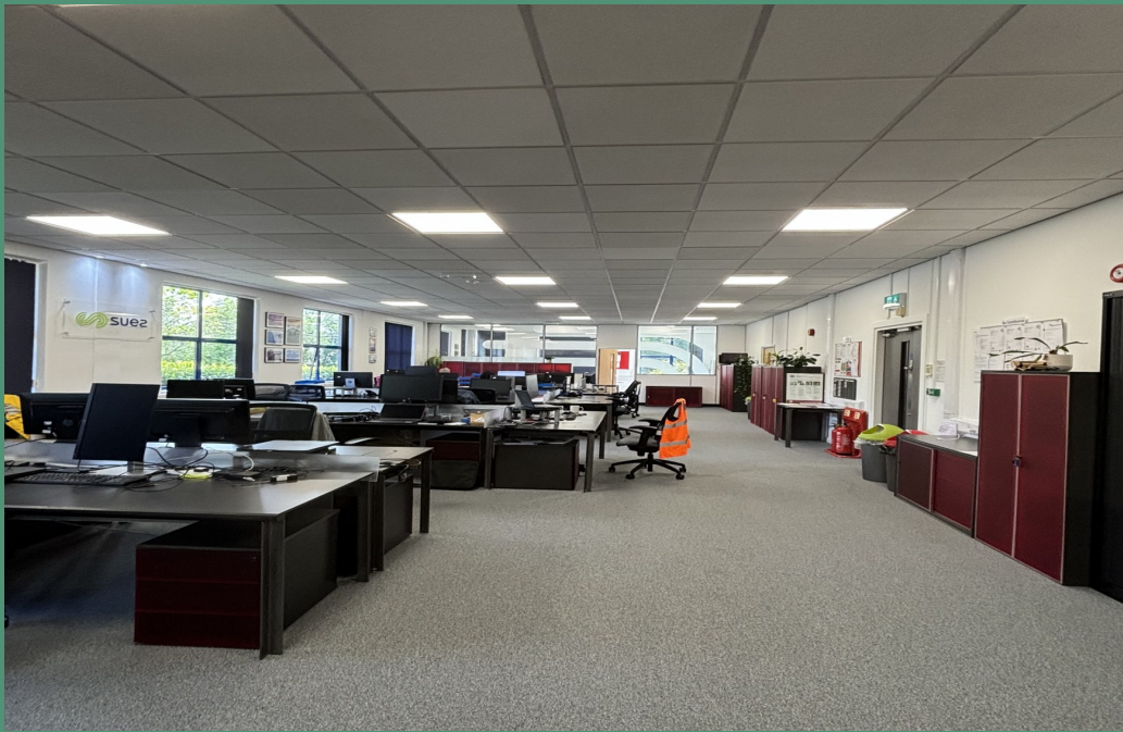
OFFICE SPACE CURRENTLY BEING REFURBISHED
